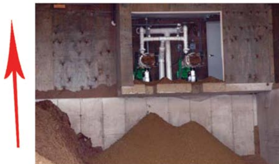
The Byproducts —After the gas has been removed, the water is removed, leaving the best bedding available for the cows. The process starts all over again, with the bedding and manure getting mixed together.
