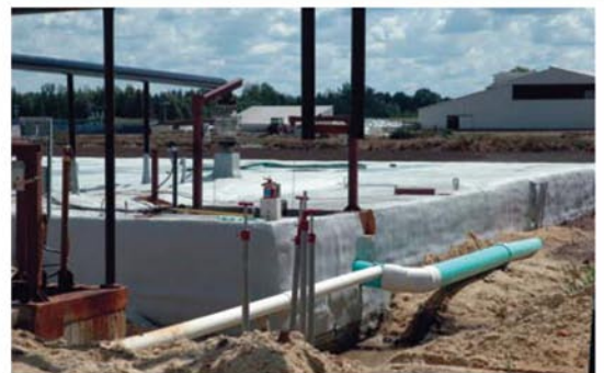
The Storage Pit —The manure enters in here and flows through channels in the enclosed pit. It takes 21 days from entering to when it exits to produce the methane gas.
